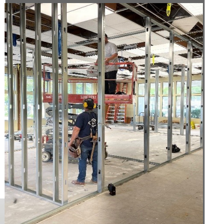
830 College Avenue Tenant Improvements
