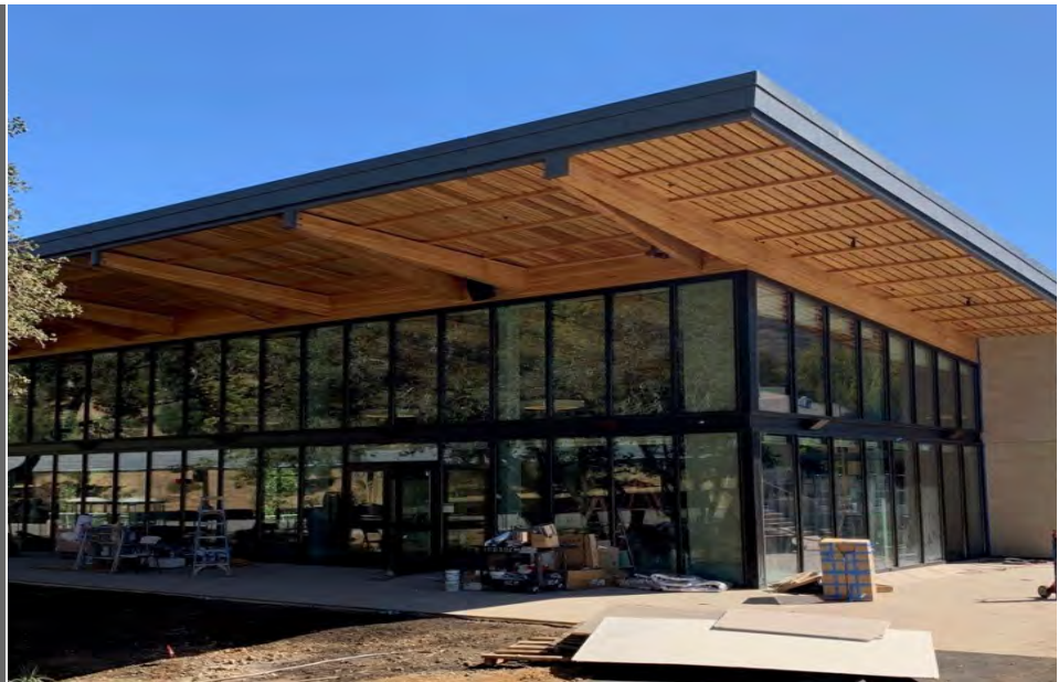
Bill and Adele Jonas Center Construction, Indian Valley Campus
