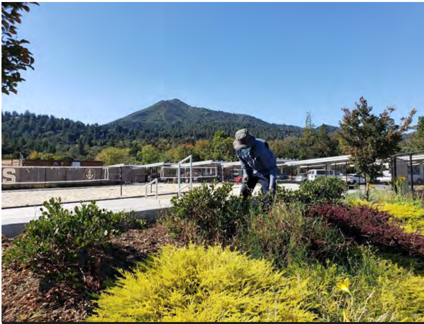
Landscaping in progress at Kentfield Campus
