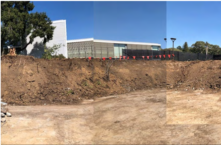
Demolition of Learning Resources Center, Kentfield Campus
