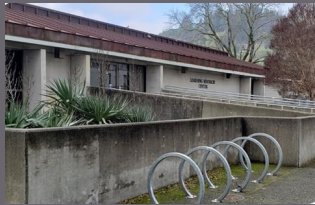
Demolition of existing and construction of new Learning Resources Center building
