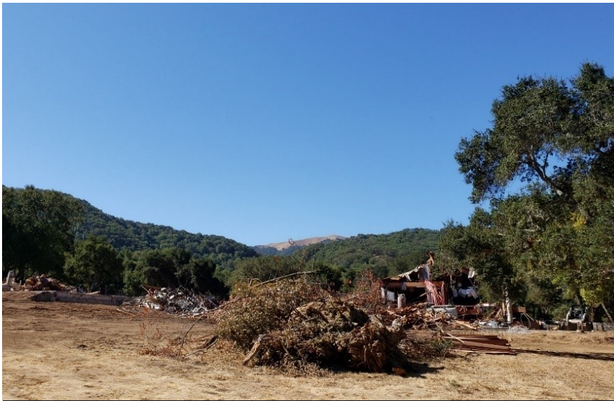
Miwok Cluster Demolition, Indian Valley Campus
