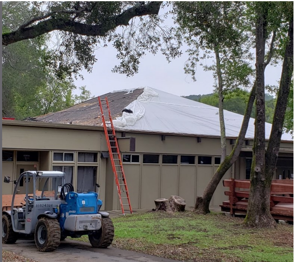
Admin Cluster & Building 12—Roof Replacement, Indian Valley Campus
