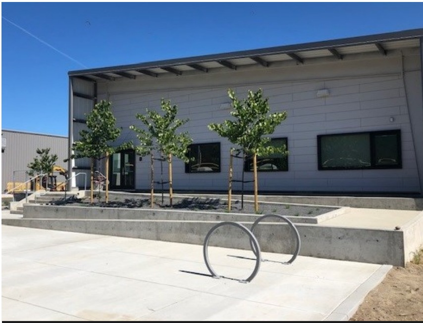
Main Entrance of the new Maintenance and Operations Building at Kentfield Campus
