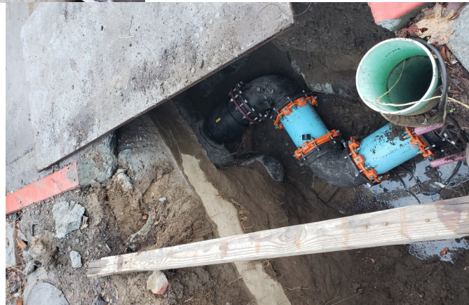
Geothermal Water Line Repair at Kentfield 2018
