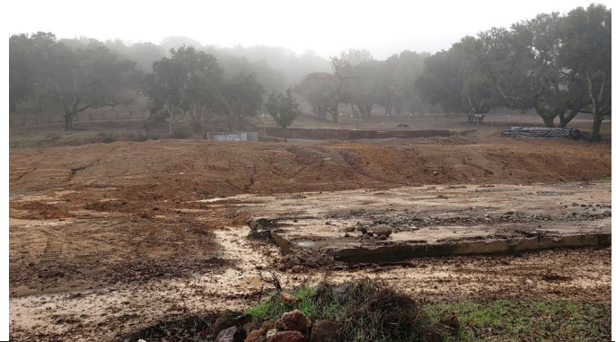
Miwok Cluster—Site Work, Indian Valley Campus
