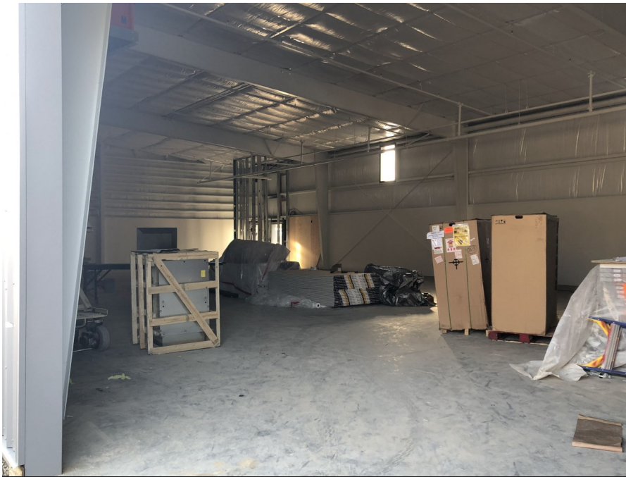
New District Warehouse Construction, Kentfield Campus
