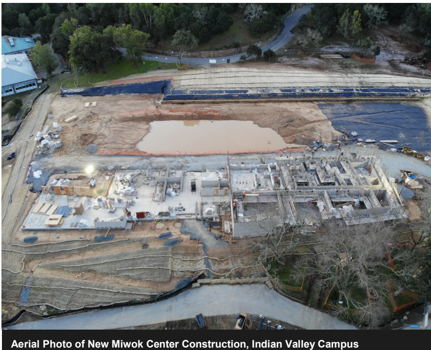
Aerial Photo of New Miwok Center Construction, Indian Valley Campus
