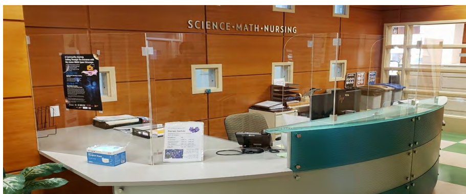
Safety Shield Installation at Science Math Nursing, Kentfield Campus
