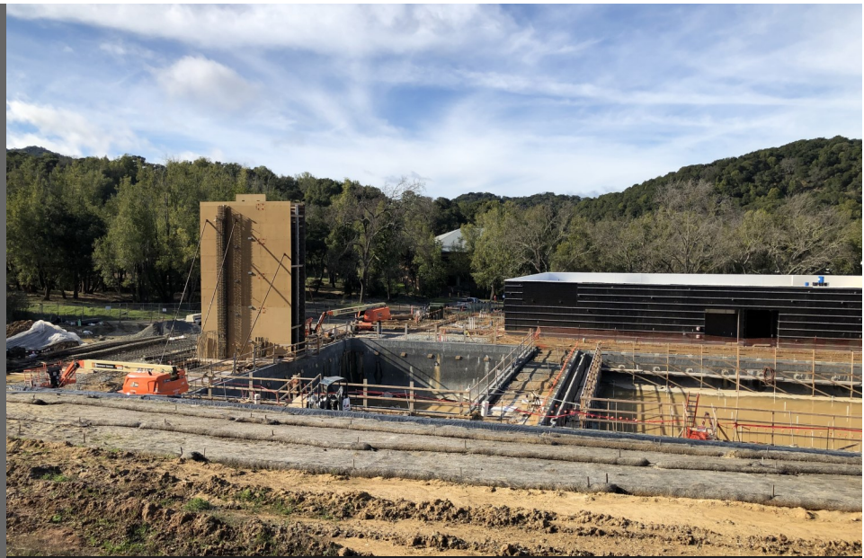
New Miwok Center Pools and Dive Tower Construction, Indian Valley Campus
