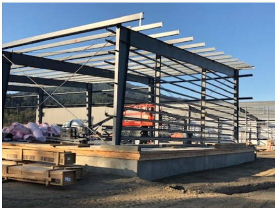
Maintenance and Operations Building, Kentfield Campus
