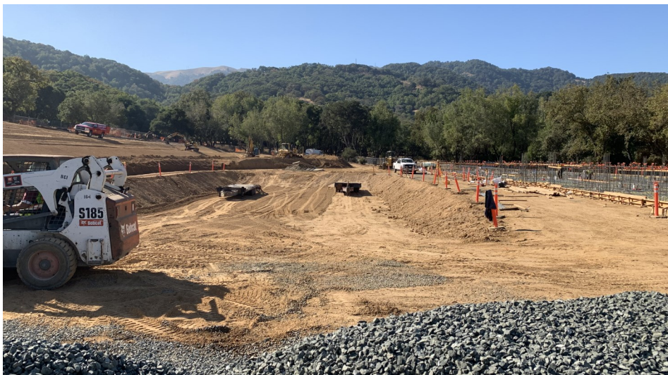
Pool Excavation of New Miwok Center, Indian Valley Campus
