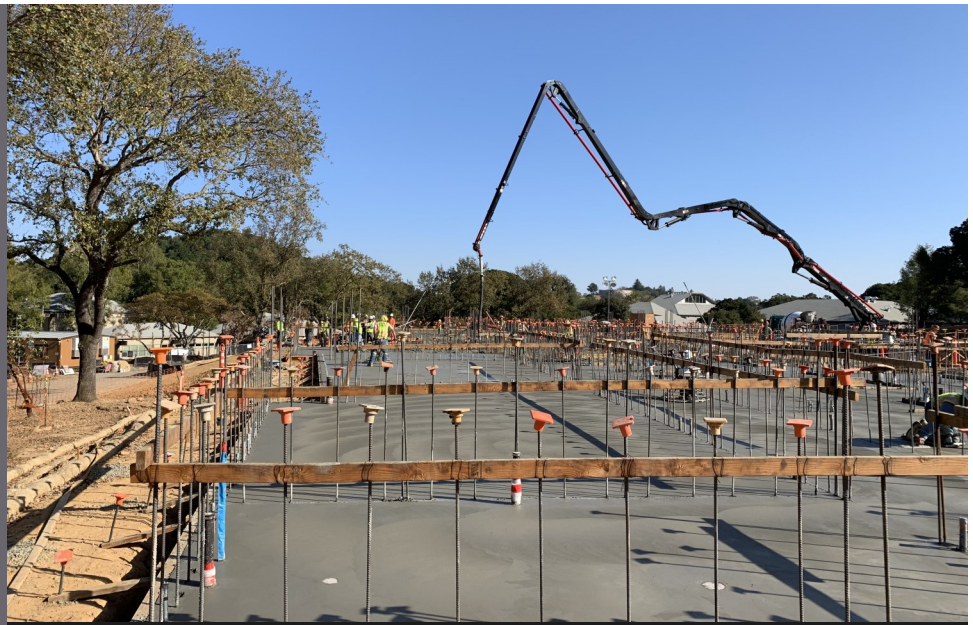
New Miwok Center Slab Placement, Indian Valley Campus
