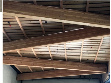
Bill and Adele Jonas Center construction, Indian Valley Campus
