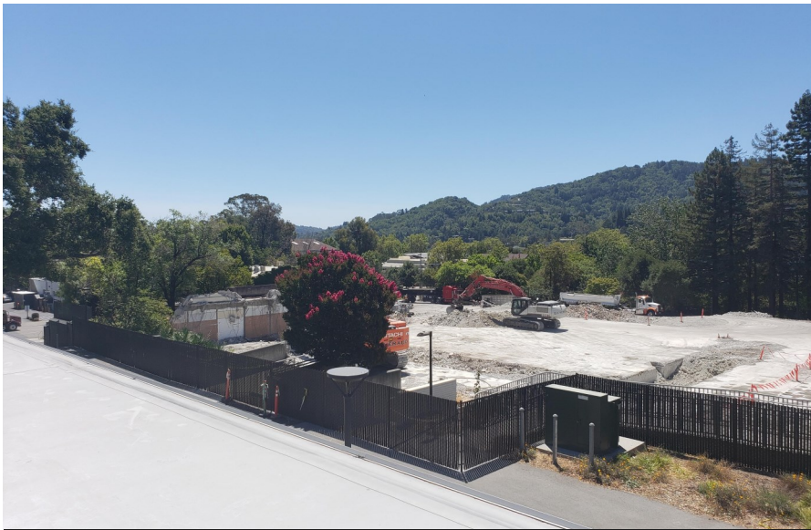
Demolition of Learning Resources Center, Kentfield Campus
