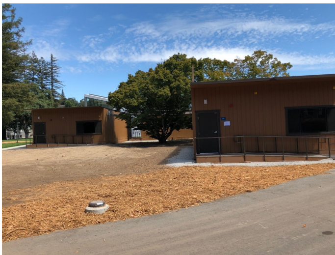
Relocated Portables at Kentfield Campus
