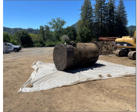
Underground Storage Tank, Learning Resources Center, Kentfield Campus
