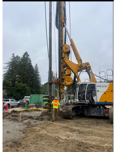
Deep Cement Soil Mixing, Learning Resources Center, Kentfield Campus
