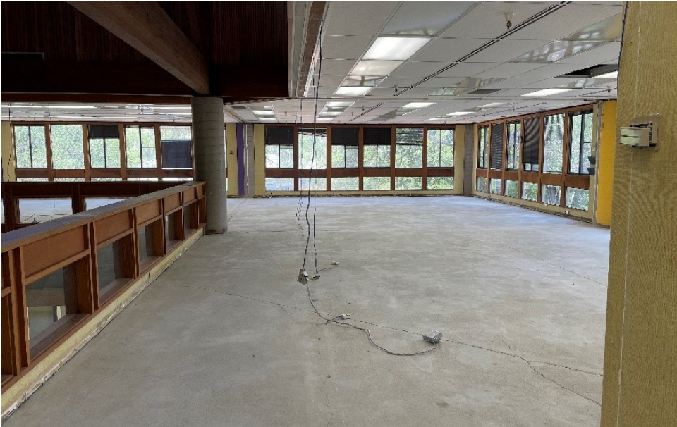
Summer Project: Abatement and Interior Demolition of Building 17 at Indian Valley
