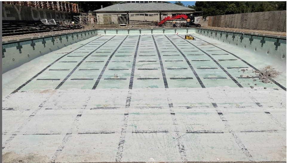
Summer Project: Old IVC Pool Demolition
