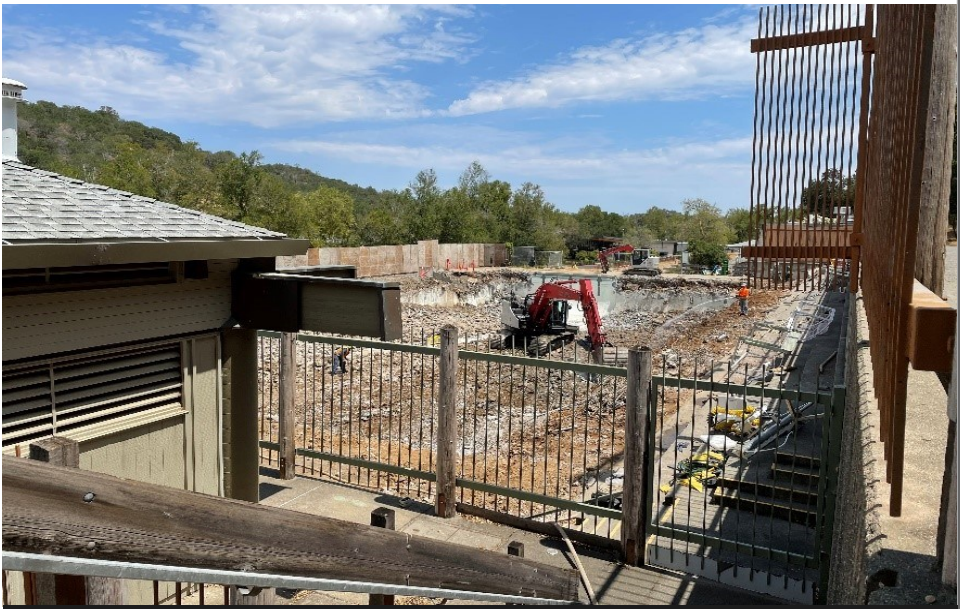
Summer Project: Old IVC Pool Demolition
