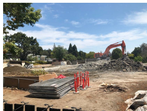
Learning Resource Center Demolition, Kentfield Campus
